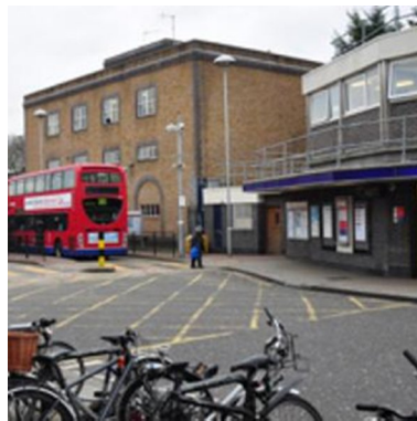
Photo 14: Northern station entrance
