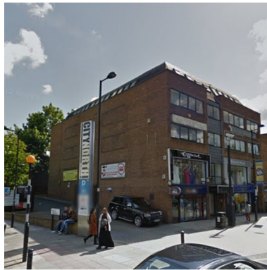
Photo 13: City North site
