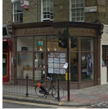
Photo 29: Locally listed building
