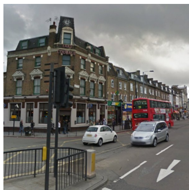
Photo 19: Intact historic block
