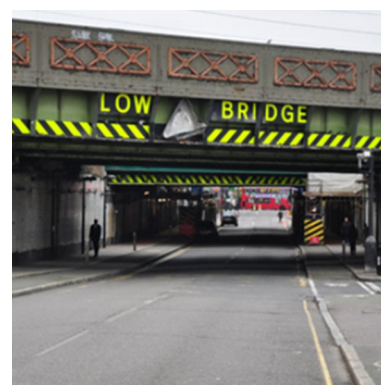
Photo 12: Bridge, Stroud Green Road
