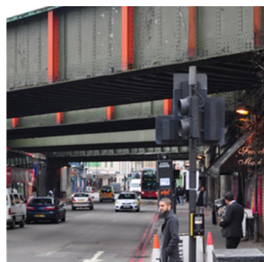
Photo 22: Seven Sisters Road viaducts
